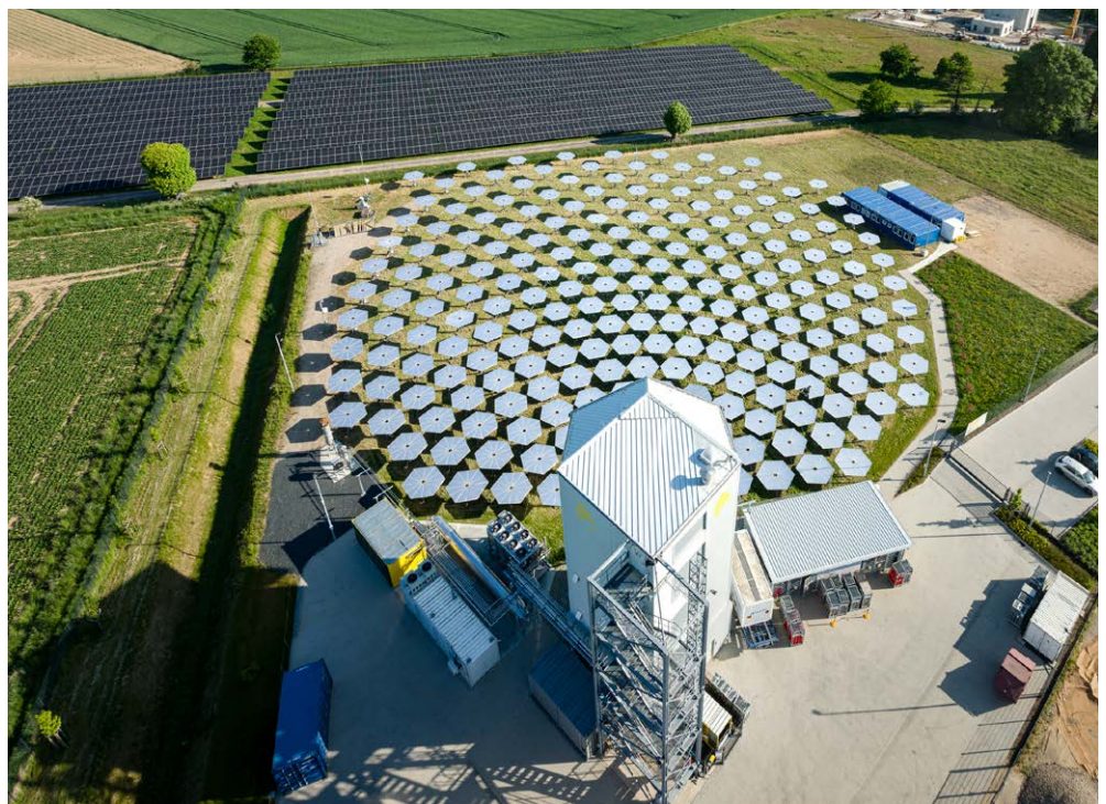
At this facility in Germany, Synhelion produces synthetic fuel using sunlight and CO 2 (Photo: Synhelion)
