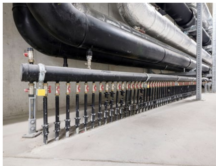
Energy piles are already in use for the Circle.
