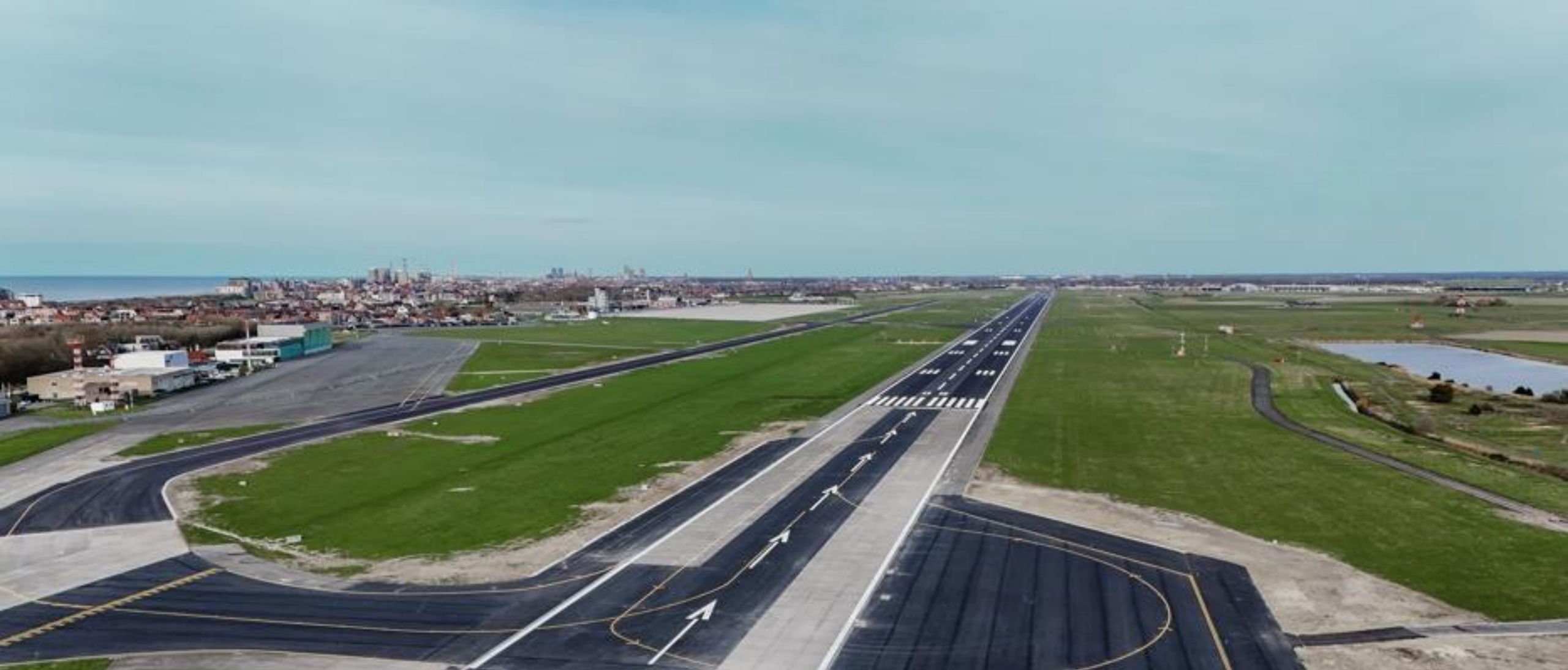
Airside infrastructure -Runway renovation (25 January-29 March 2024)
